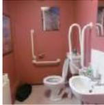
**18.7** Bussage Primary School has one disabled toilet located in the men's facilities. It has been adapted and not specially built. The walls provide a good contrast to the fittings. It does not have an alarm which is recommended, the mirror and coat hooks are too high for a wheelchair user, there is no grab bar on the back of the door and it is cluttered.
